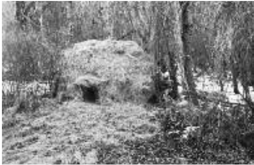
Architect Gáyor's Soft House, 1971
